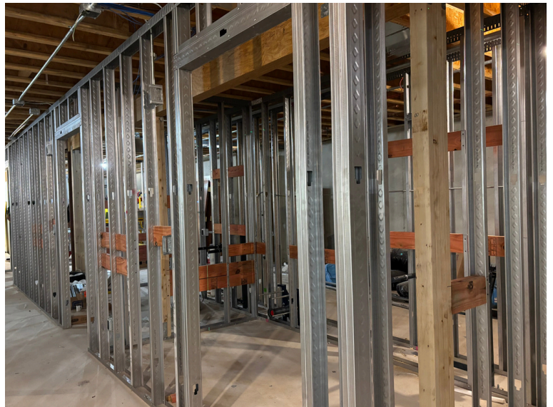
Metal framing for bathrooms on the lower level.
